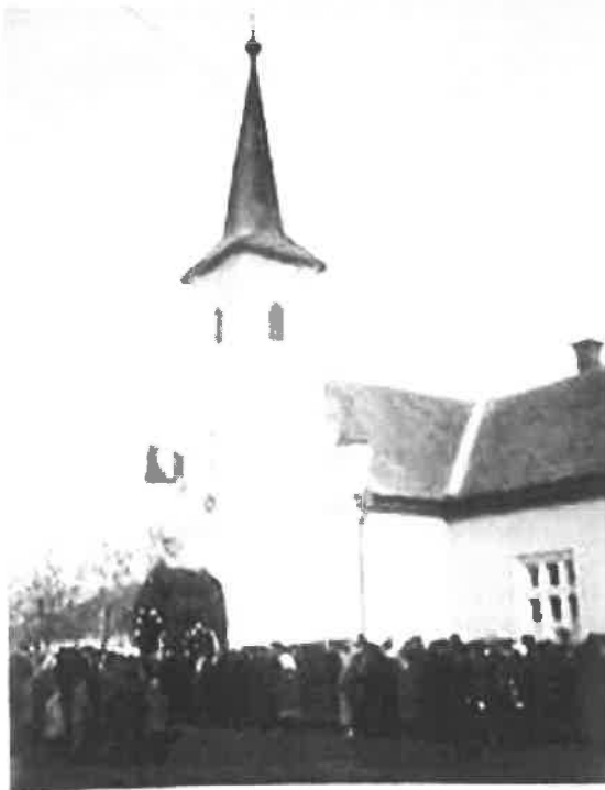
A more detailed investigation of the following conditions would be desirable.
